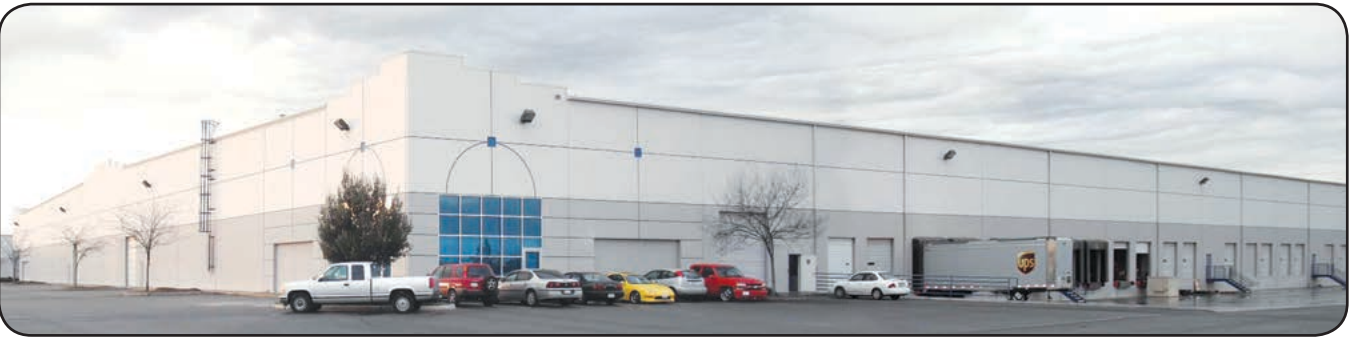
Fresno, CA Warehouse facility; 100,000 sq. ft.
