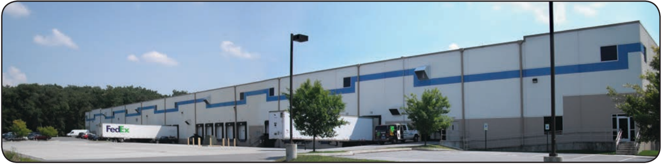
Elizabethtown, PA Warehouse facility; 144,000 sq. ft.
